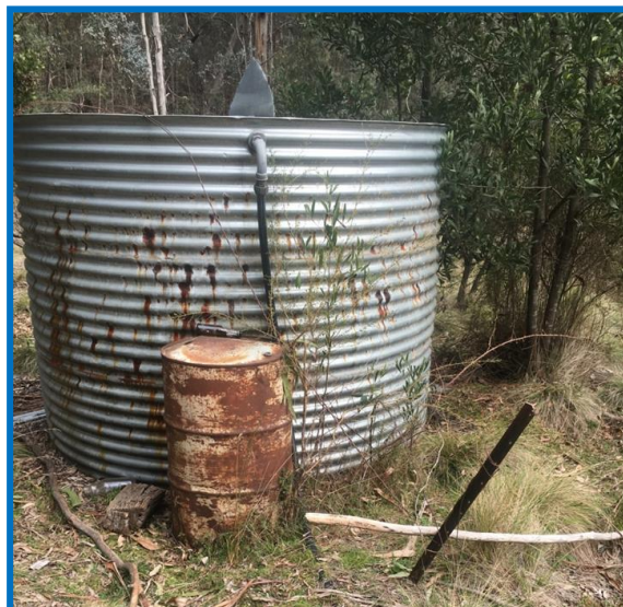
Redundant Mirimbah Store Buffer Tank
