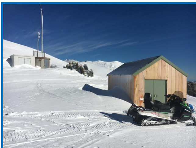
New High Level Water Treatment Plant Building
