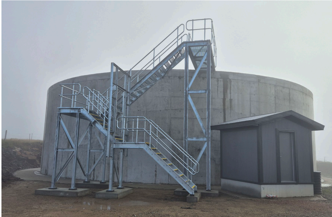
Figure 9: The Higgi Tank Access Stairway.
