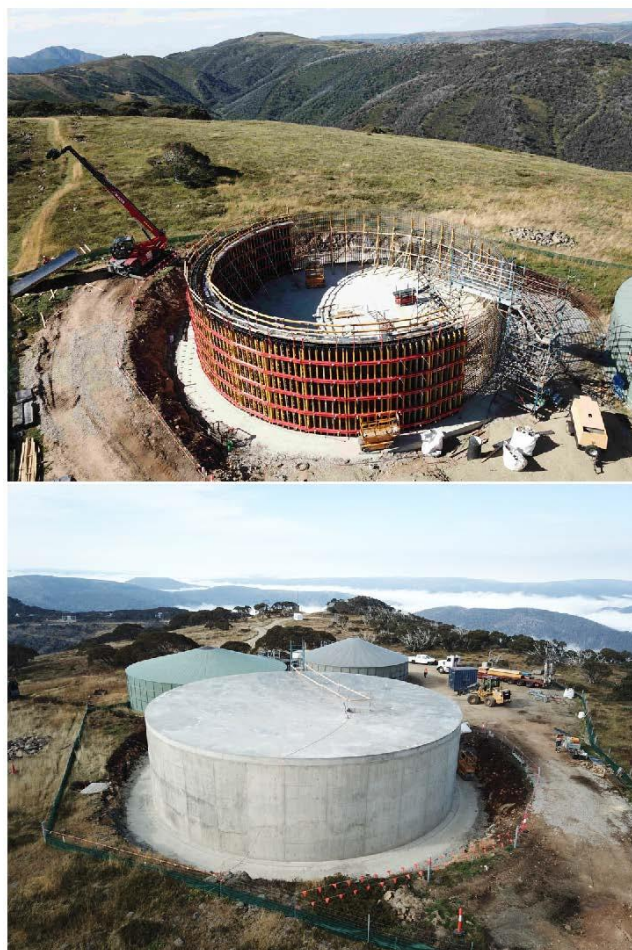
Figure 9: New 2.2ML Mt Higgi Raw Water Storage Tank
