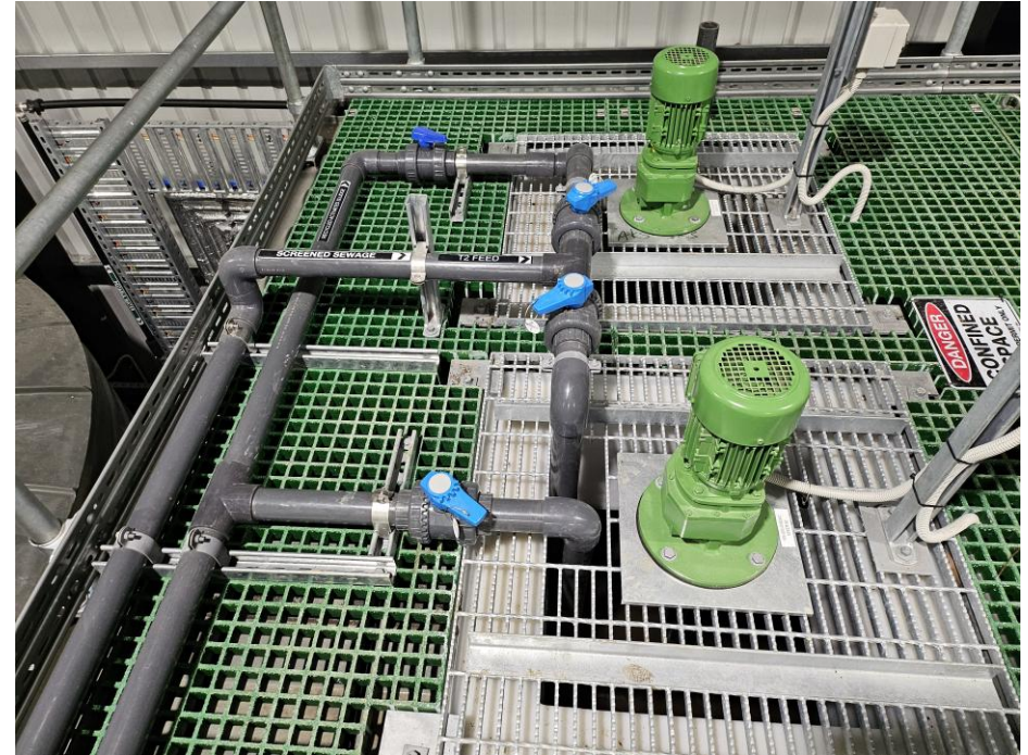
Figure 7. Inside the wastewater treatment plant
