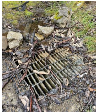
Maintenance of pits and pipes is important.
