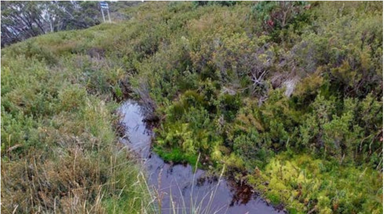
Photo 16 Aqueduct between Bog 11.2 (right) and Bog 12 (left), facing east (IY2; 25 February 2021, after construction).
