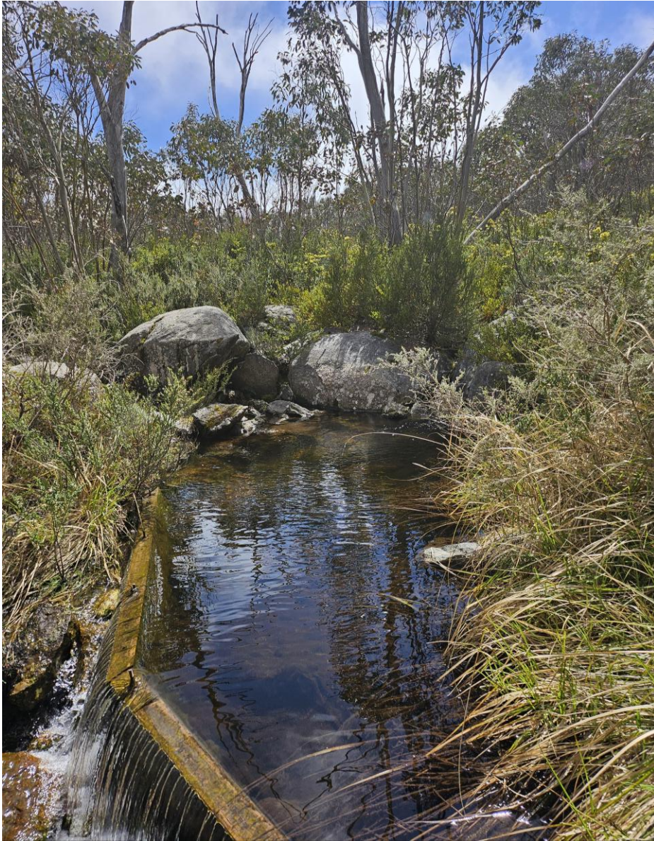
Figure 15. Taggerty River weir diversion for use in the resort for potable and snow making uses.
