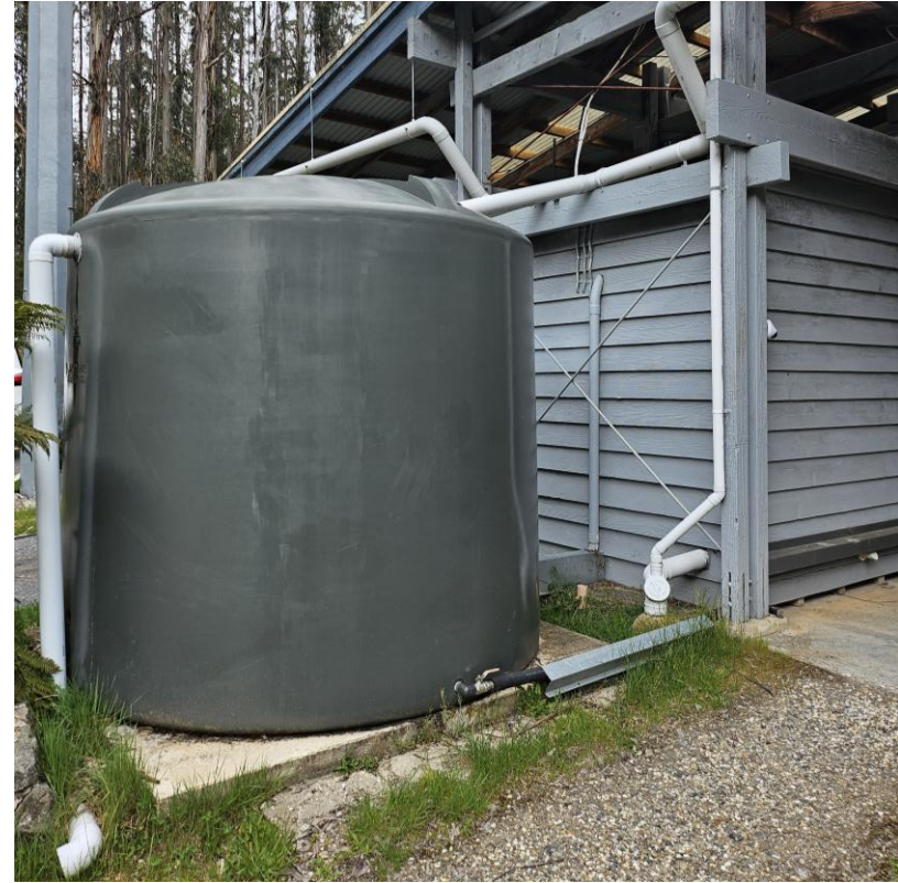
Figure 9. Photo of tank at resort entry
