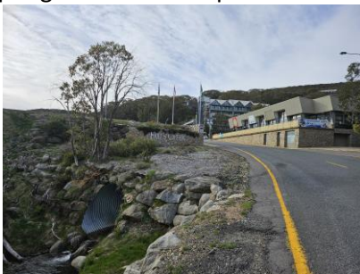
Maintenance of pits, pipes and outlets is important.
