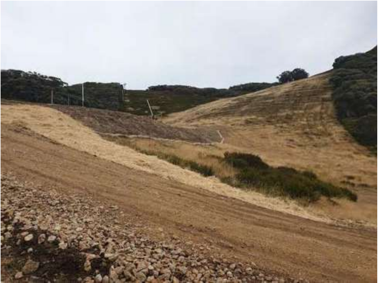
Photo 11 Earthworks surrounding Bog 13 in IY4 (IY4; 25 May 2023)
