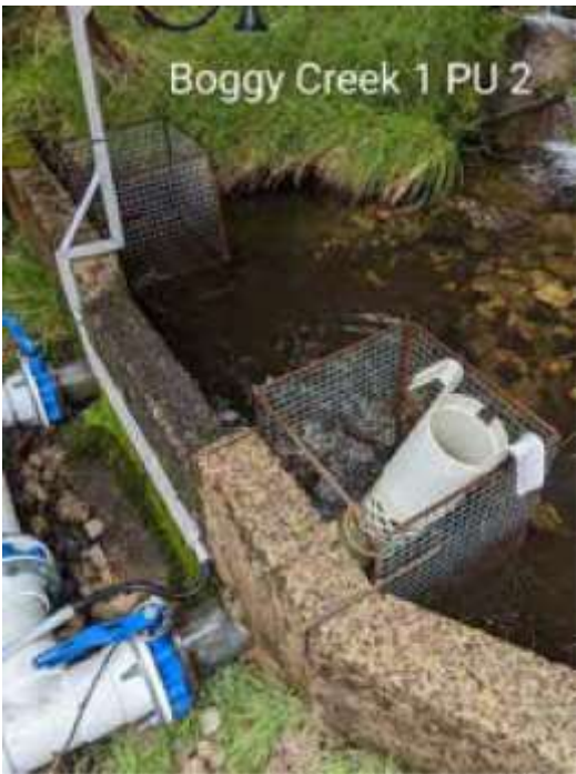
Figure 3 Boggy Creek 1 PU 2 location
