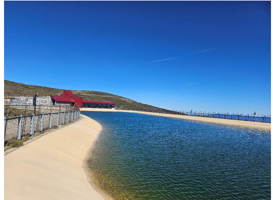
Figure 11. Loch Dam at near full supply (Source: Wave Consulting Australia)
