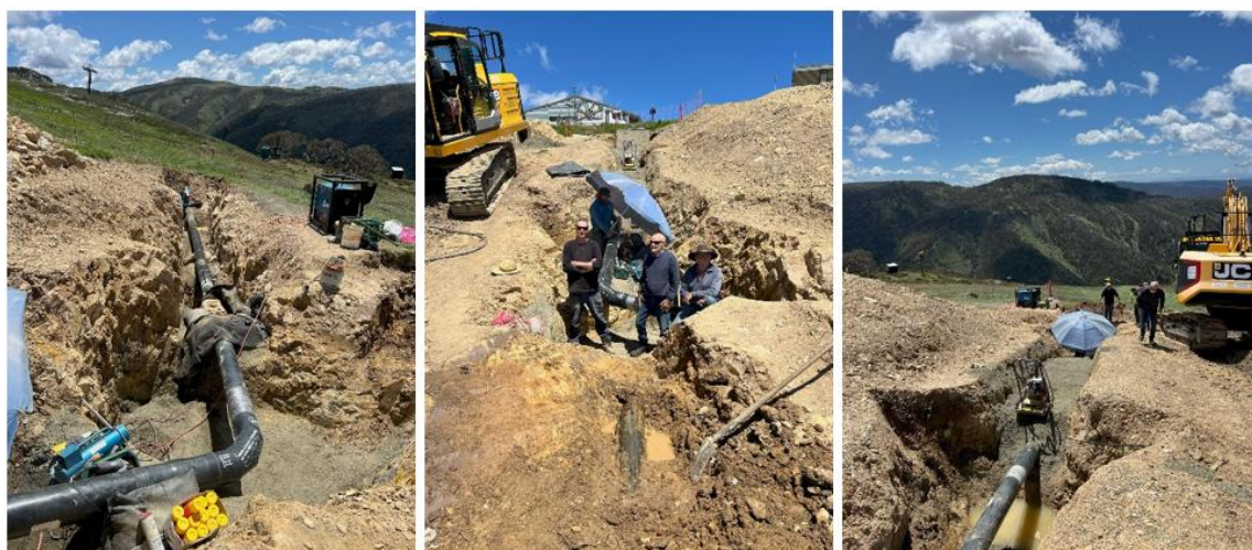
Figure 9: Final Section of Raw Water Rising Main Replacement Project
